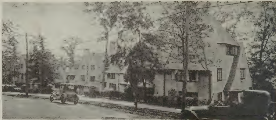
VIEW LOOKING SOUTH, OAK COURT TERRACE DEVELOPMENT
